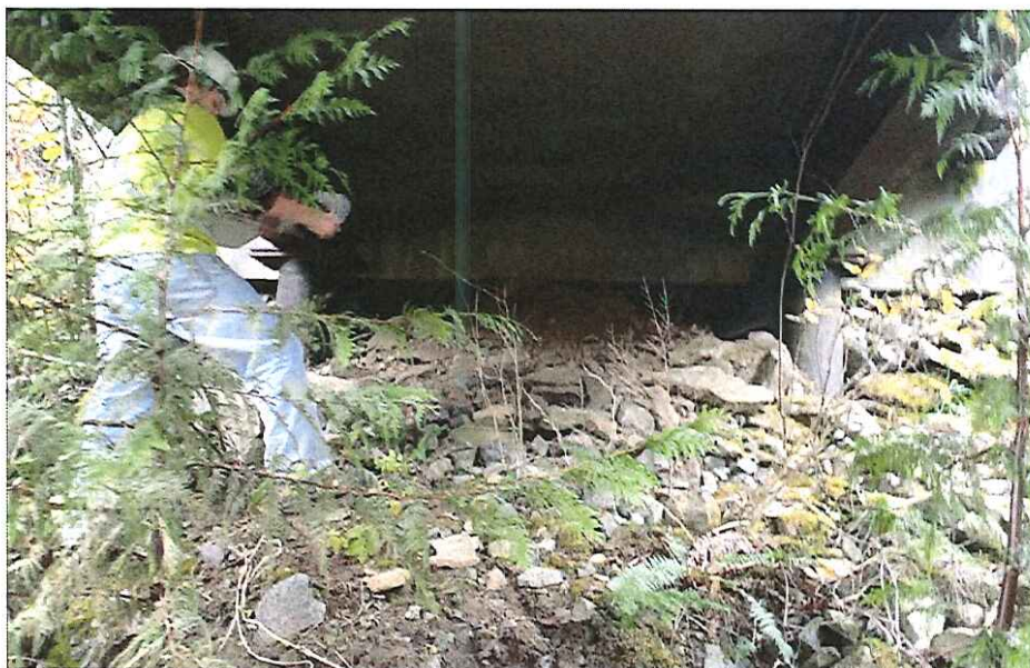
CK2395 Right Abutment2
