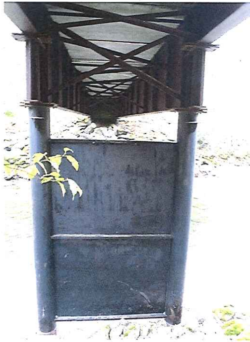
CK2395 Pier from Right
