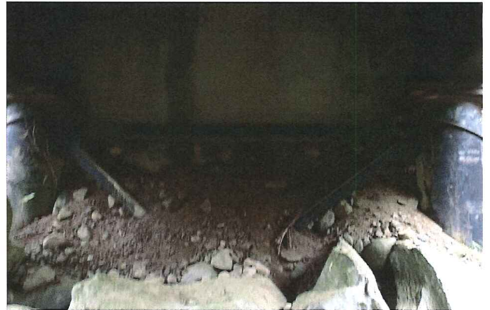
CK2395 Left Abutment
